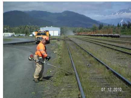
Mechanical control in Seward Yard is not effective in meeting vegetation management requirements.
