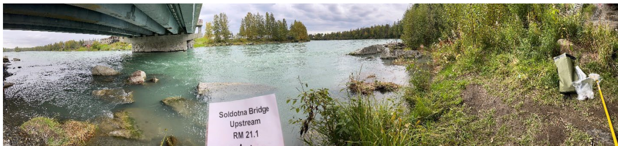
Figure A. 9. River mile 21.1 looking northeast. Photo collected in September 2022.
