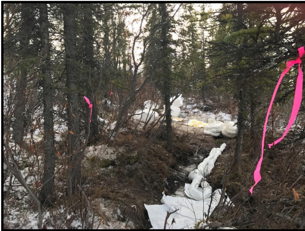
Spill site with hydroexcavated trench containing sorbent material, on November 13, 2016. (Photo/BLM)
