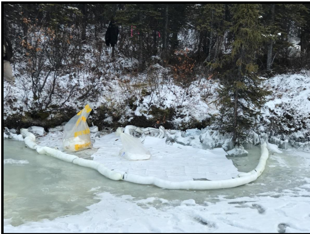
Affected area of Paxson Lake with absorbent boom and pads to recover migrating product. (Photo/BLM)
