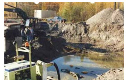
Excavation of large underground storage tank on base.
