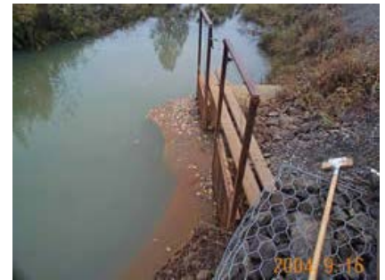
Gates in Garrison Slough which prevent the passage of fish into and out of the contaminated reach of the slough.
