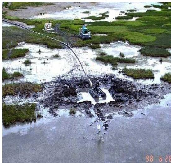
Pump placed in pond to dry out sediments to render white phosphorus harmless.
