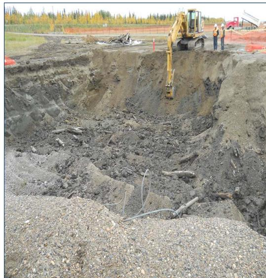
Air Force contractors excavated 8,700 cubic yards of petroleum-contaminated dirt in the summer of 2013 as part of an Interim Removal Action for site SS016 at the northern edge of a Galena Airport runway. The soil was taken to the Galena landfarm on the Campion Airstrip. An Interim Removal Action is an interim measure to remove or isolate contamination any time during the cleanup process to protect people and the environment. (DEC photo)
