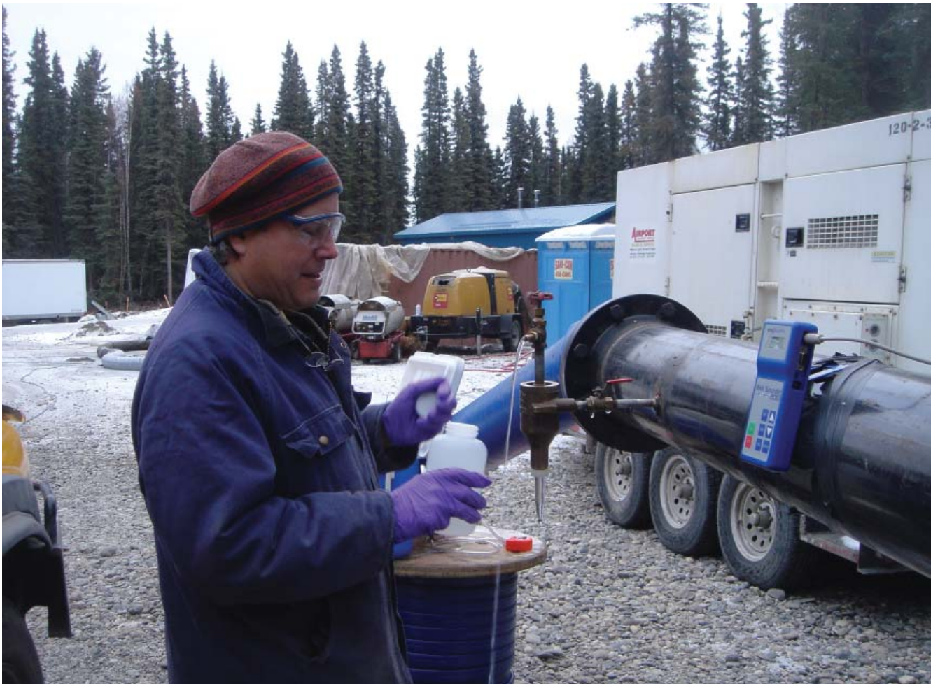
Shannon & Wilson Inc.'s Mark Lockwood collects a sample for the new City of North Pole distribution wells last October. Shannon & Wilson is a Flint Hills contractor. Photo courtesy of Shannon & Wilson.
