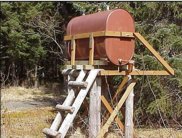
Check for tank stability. Legs for tanks should be resting upon a solid foundation. The bottom of the tank should be off the ground and clear of debris.
