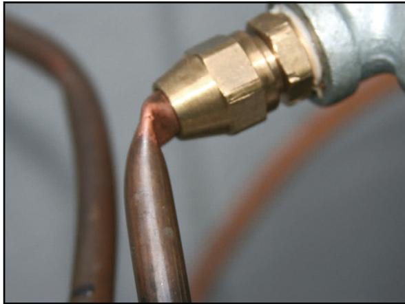
Check fuel lines to make sure they are not damaged or leaking. Pay close attention to connections or joints which can fail.
