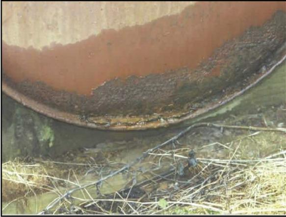
Replace your tank if it is rusting or if the tank appears damp! Painting tanks with a rust inhibitor paint will prolong the life of your tank.
