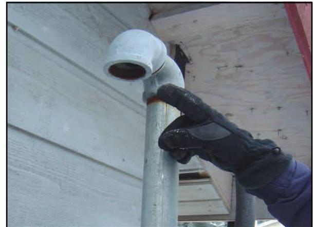
Check the tank vent for any obstructions like snow, ice, insects or spiders.
