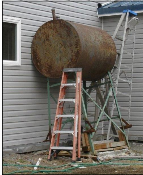
The set up of this tank makes it very vulnerable to damage from an earthquake or a flood.
