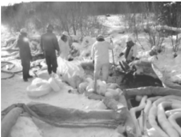
Placing sausage boom in creek, on west side of tracks.
