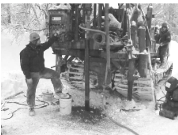
Rig used to drill sentinel wells.
