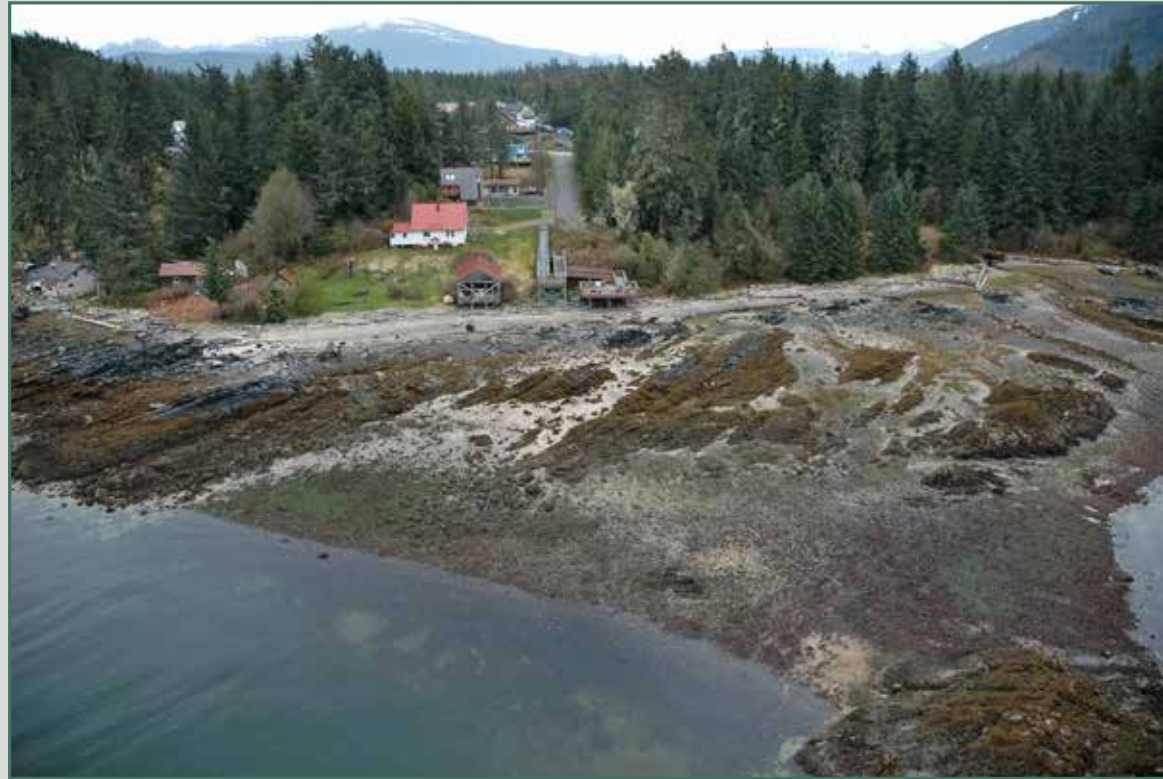
DF01 viewed from the west.
