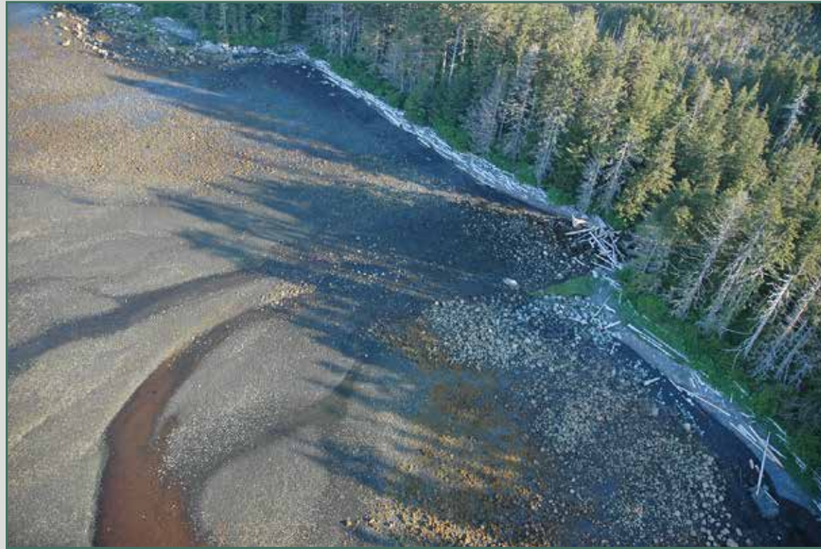
EX01d viewed from the southeast.
