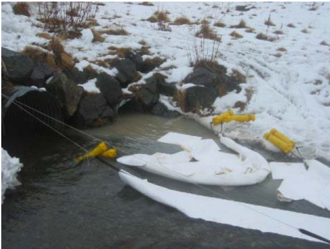
Culvert outfall with sorbents deployed (photo courtesy USCG MSD Dutch Harbor)
