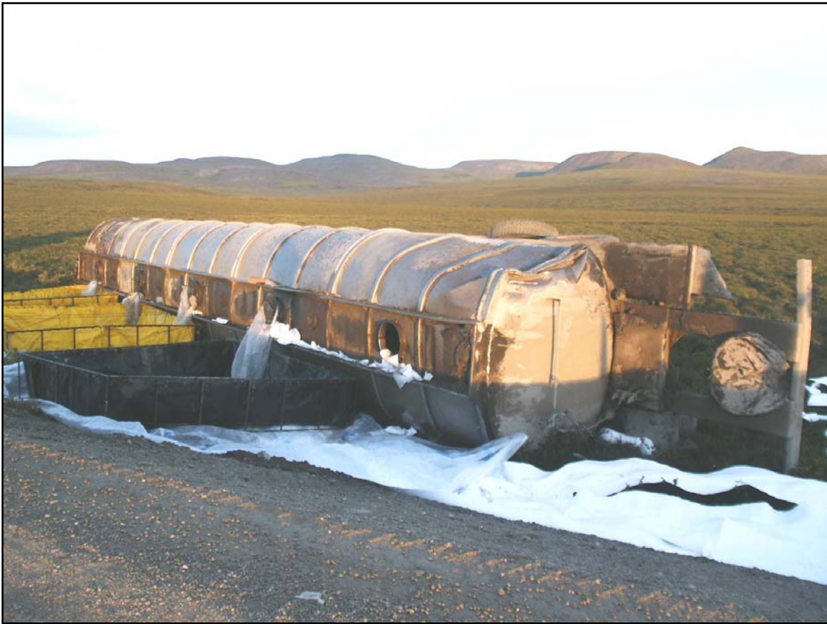
Photograph courtesy of TeckCominco - Photo shows the fast tanks setup to contain diesel spilling from the overturned tanker.
