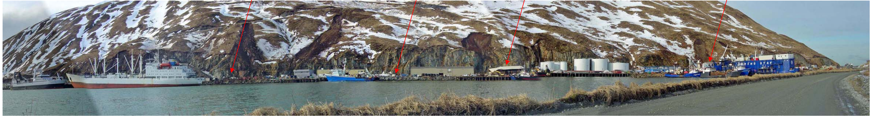
Panoramic view of the Ballyhoo Road showing the mudslide impacted area.
