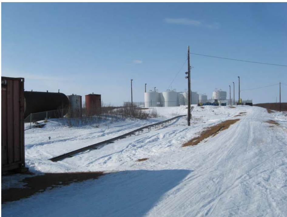
The old tank farm is the source tank of the fuel release and is located left of the photo.
