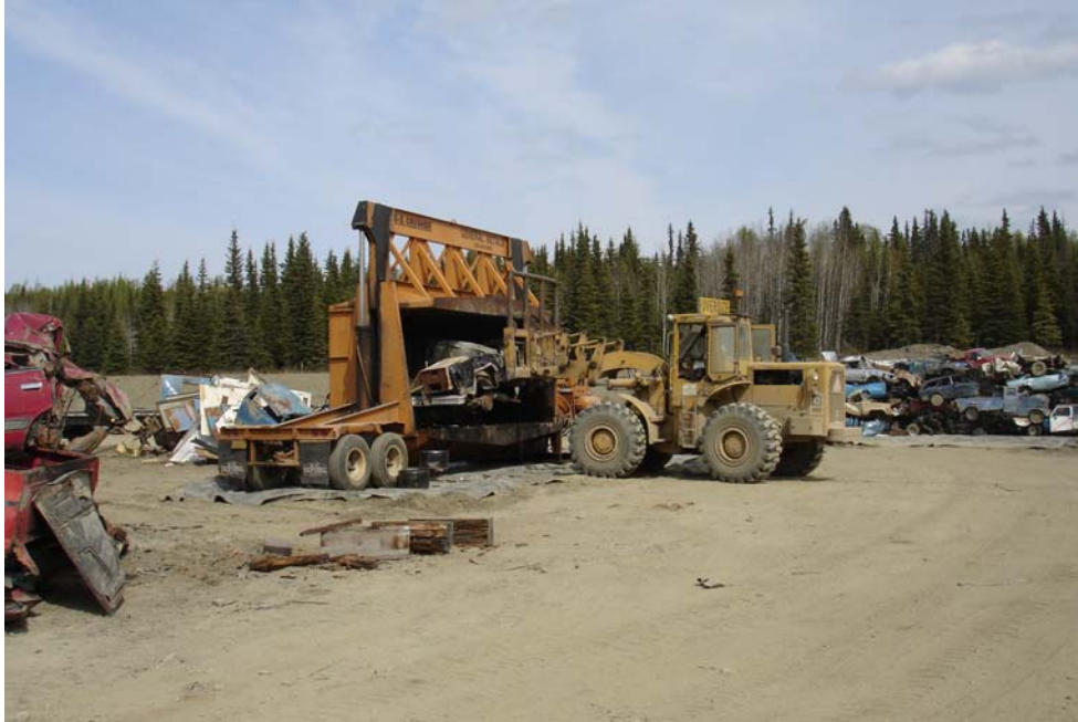
Crusher for processing vehicles for removal from site.
