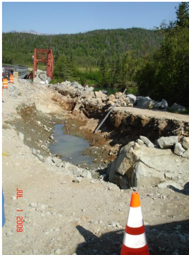
Pile Bay Road Spill Excavation Photo by ADEC
