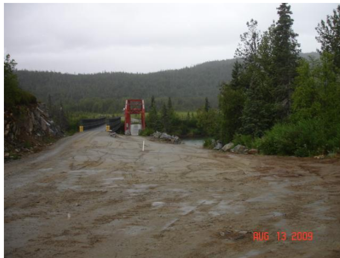
Completed Excavation Site Pile Bay Road Spill-ADEC
