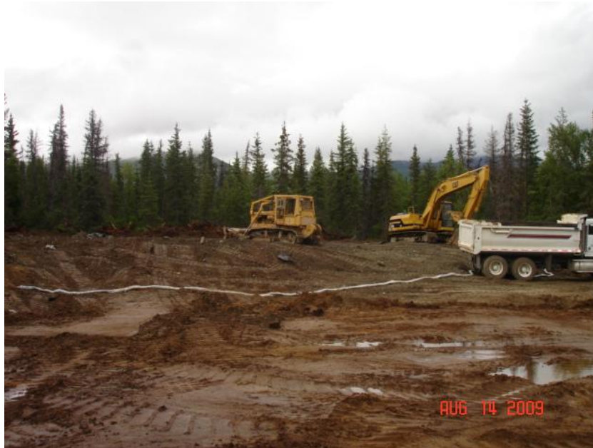
Uncompleted remediation area Pile Bay Road Spill site-ADEC
