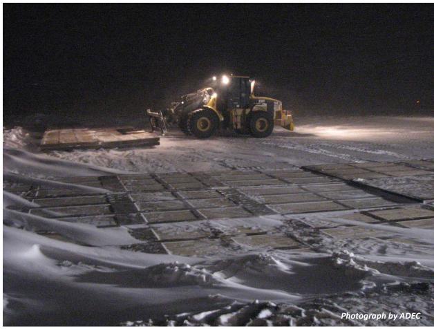
Night crews construct a 200 ft by 200 ft staging area as part of the Phase 2 spill cleanup operations. Once completed, work on a South Division machine access route can commence.
