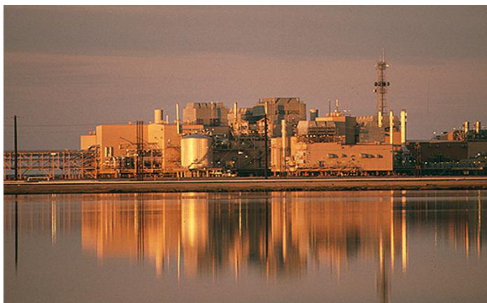
Lisburne Processing Center
