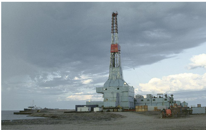
Drill rig at Point McIntyre.
