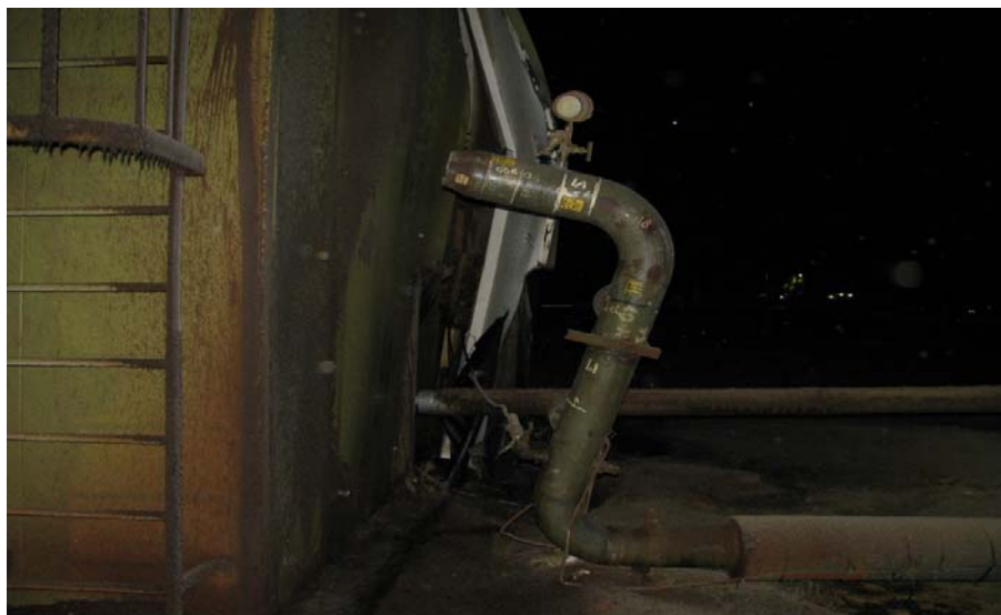
Separated 6-inch flow line
