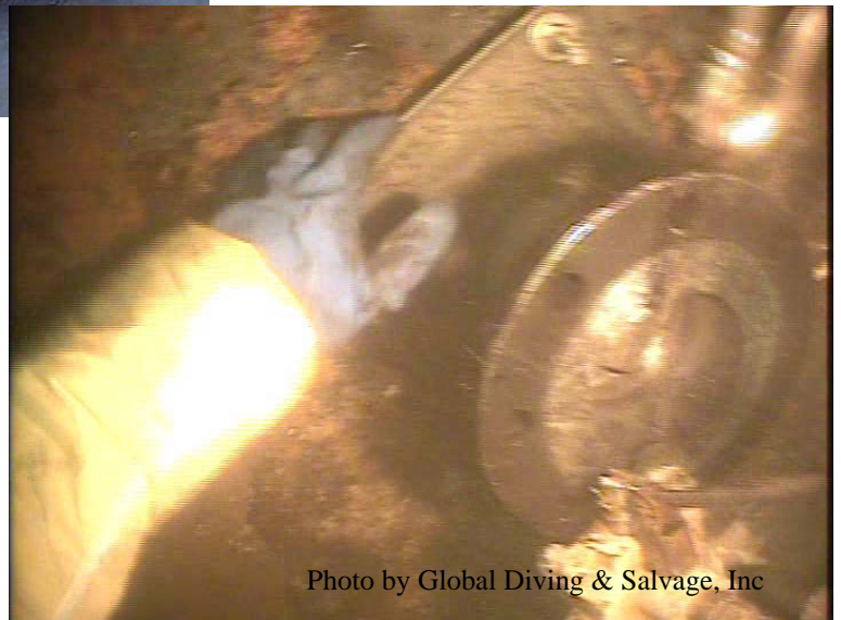
Right: Diver installing landing plates to the hull.
