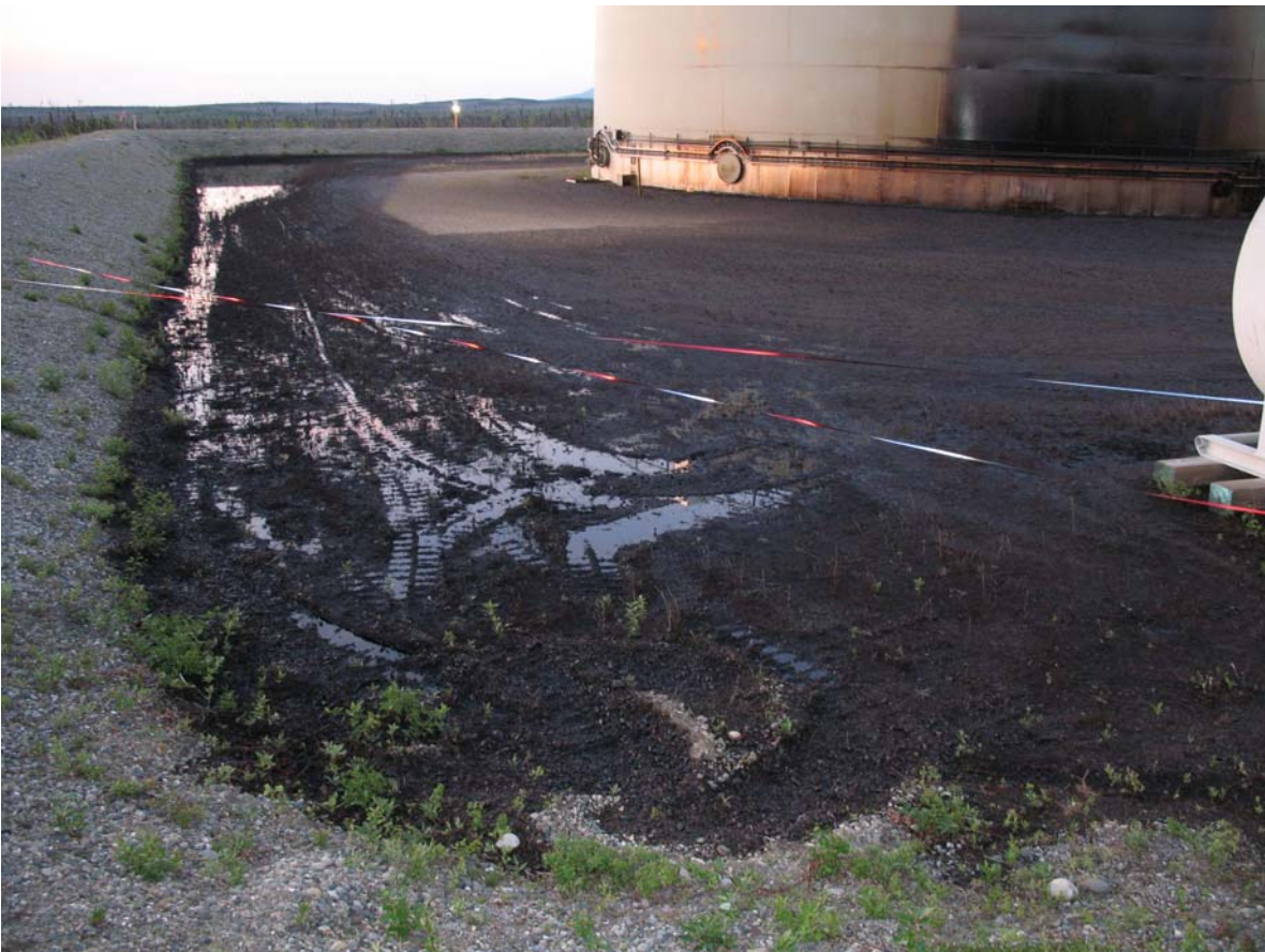
Surface of the containment area on May 28 after 36,000 gallons of oil had been drained. (APSC photo)
