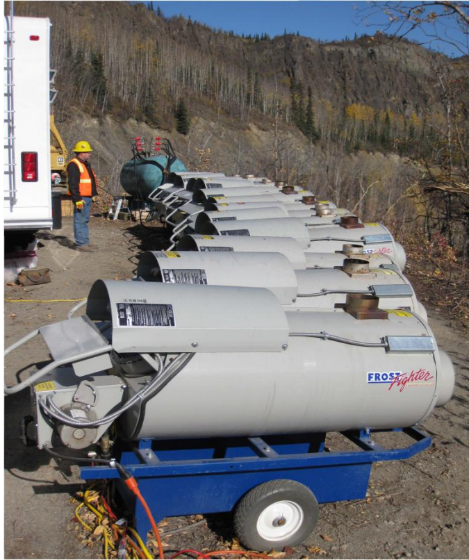
Twelve propane burners actively burning off propane, September 23, 2010. Photo by ADEC.
