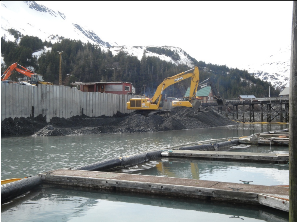
Whittier Harbor Dredging project
