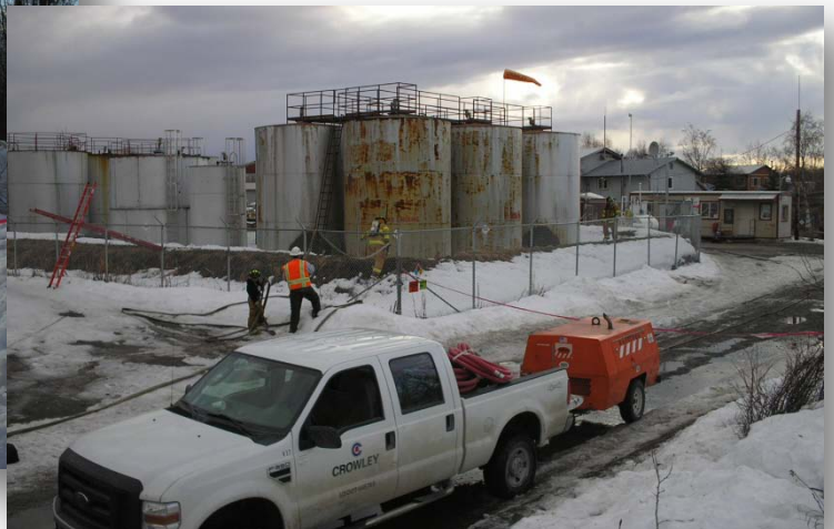
Aniak volunteer fire fighter and Crowley employees applying AFFF to reduce explosive vapors from gasoline, April 25, 2011.
