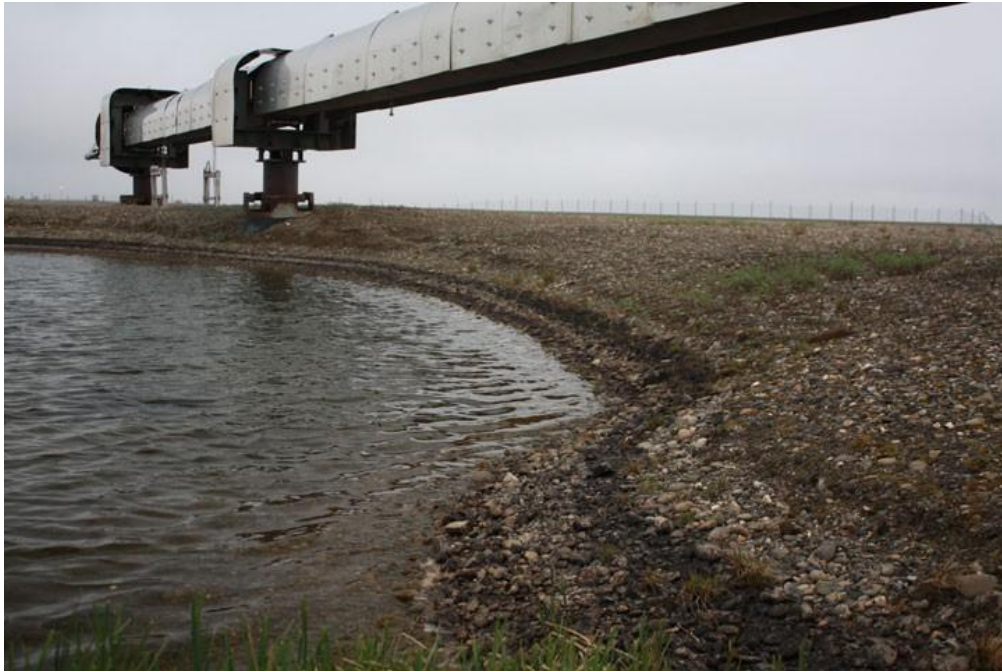
Bathtub ring surrounding the FS-2 flare pit.
