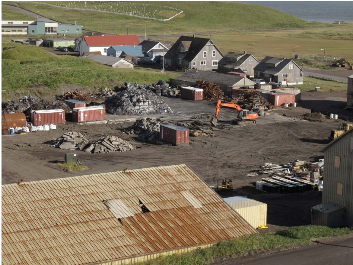
PROJECT NEAR COMPLETION, SLAB REMOVAL SEPTEMBER 22, 2012
