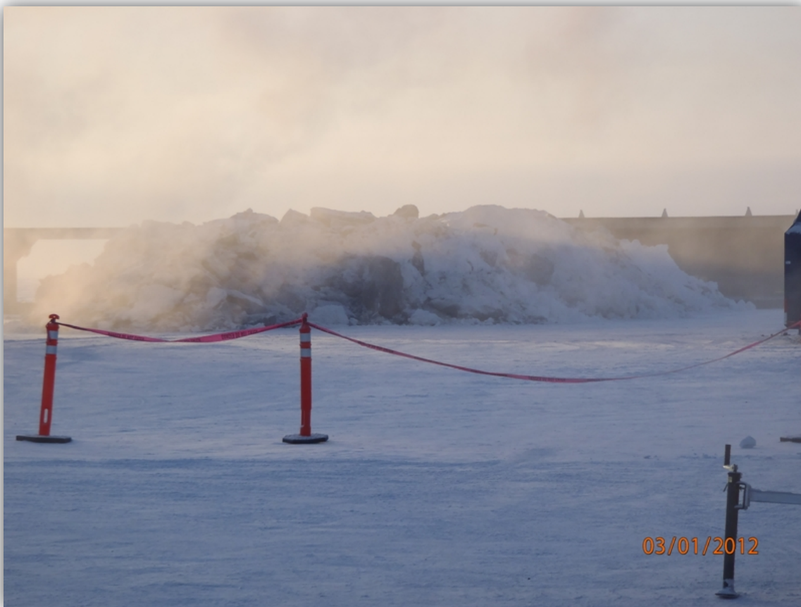
A stockpile of frozen material recovered from the pad awaits transport offsite for disposal. ADEC Photo.
