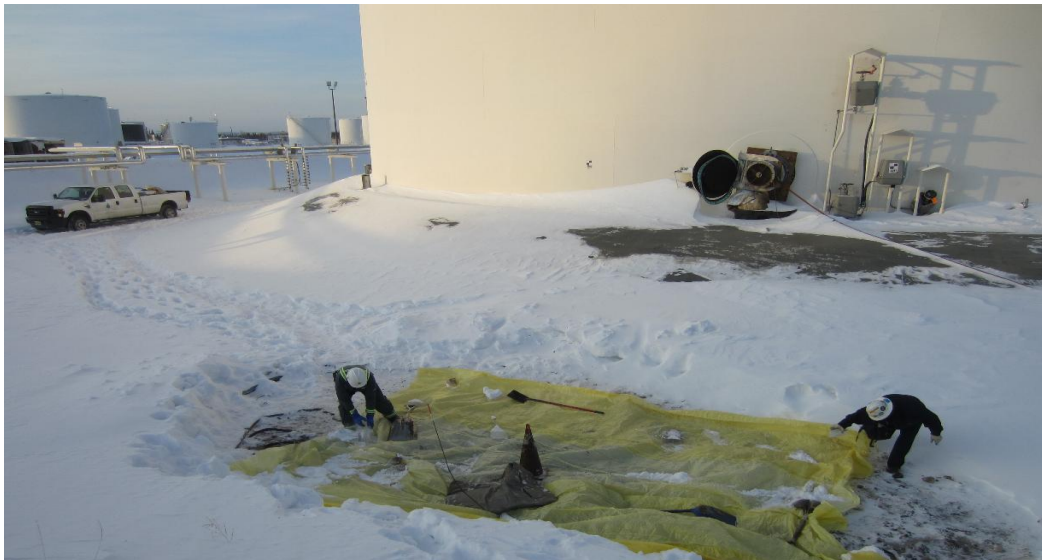
Site workers removing cover to expose spill area
