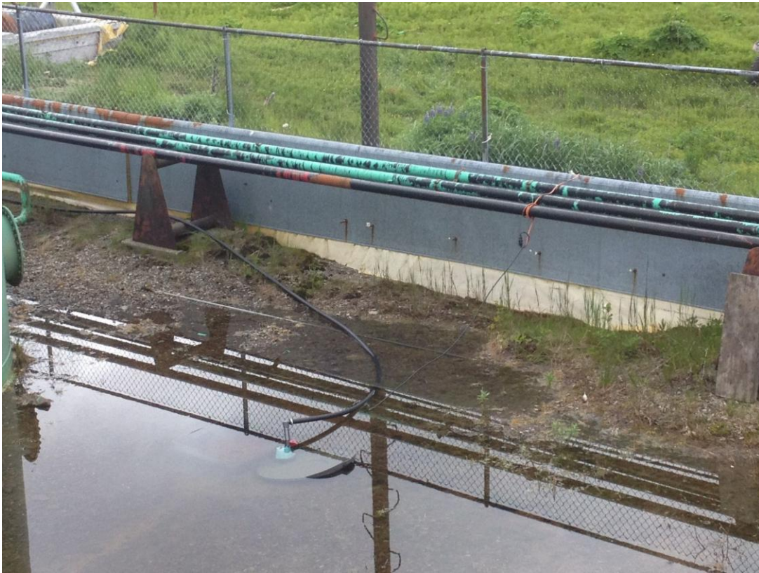
Water being drained from Peter Pan Seafoods secondary containment to be filtered. Photo provided by Peter Pan Seafoods.
