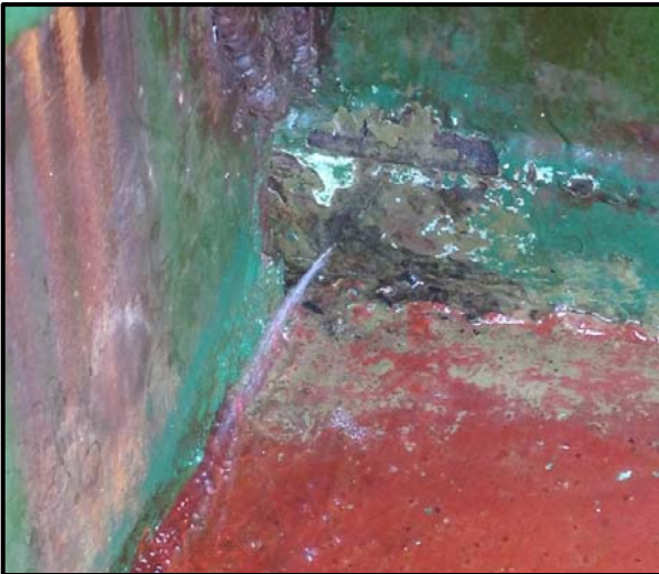
Fuel leaking through the fracture and onto the deck of the barge, September 12, 2012. (Photo/Kirby Offshore Marine)
