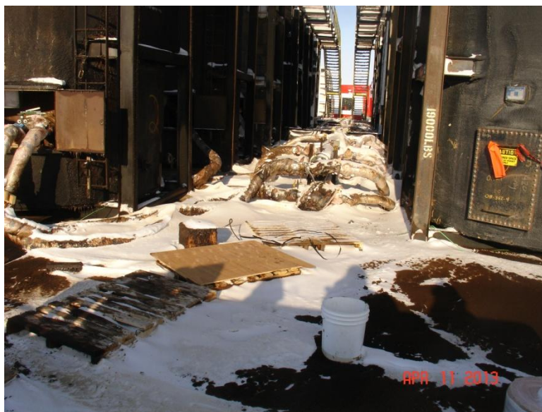
Residual fluids in the secondary containment before removal, April 11, 2013. (Photo/ADEC)
