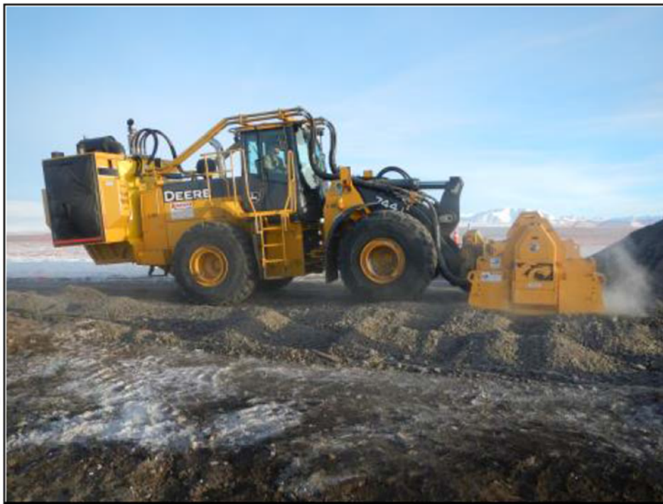
Loader trimmer working at the spill site. (Photo/ERM)
