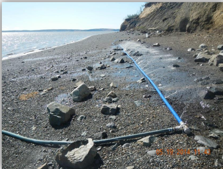
Flushing the Kakanak Beach to remove diesel contamination, May 19, 2014. (Photo/ U.S. Coast Guard)
