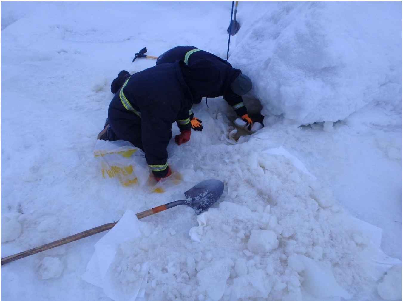
Emerald personnel recovering free petroleum product from water using absorbent pads, December 20, 2014. (Photo/Jessica Starsman, ADEC)
