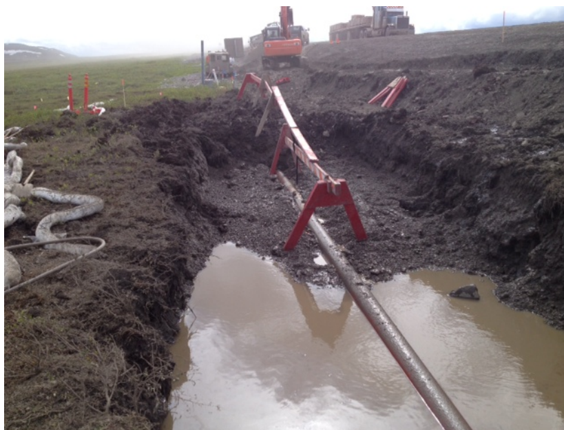
Excavation of contaminated soil along the APSC right of way. (Photo/ADEC)
