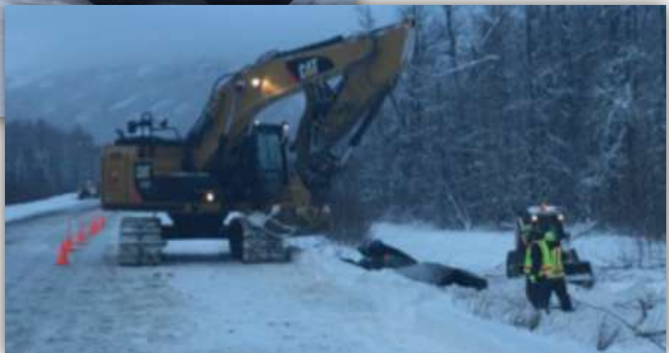
Excavating contaminated soil from the road right-of-way Photo taken 12/15/2014 by ADEC
