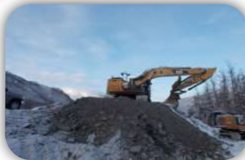
Excavating contaminated soil from the road right-of-way Photo taken 12/21/2014 by RSE
