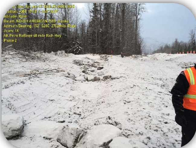
Completed site work and stream reconstruction. Photo take 01/17/2015 by ADEC
