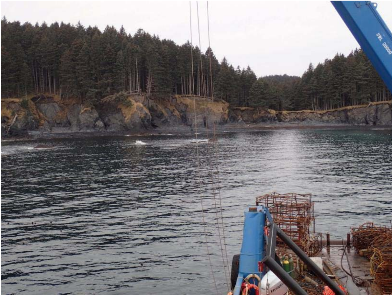
Resolve-Magone Marine Services completes debris removal, November 4, 2015. (Photo/ Resolve-Magone Marine Services)
