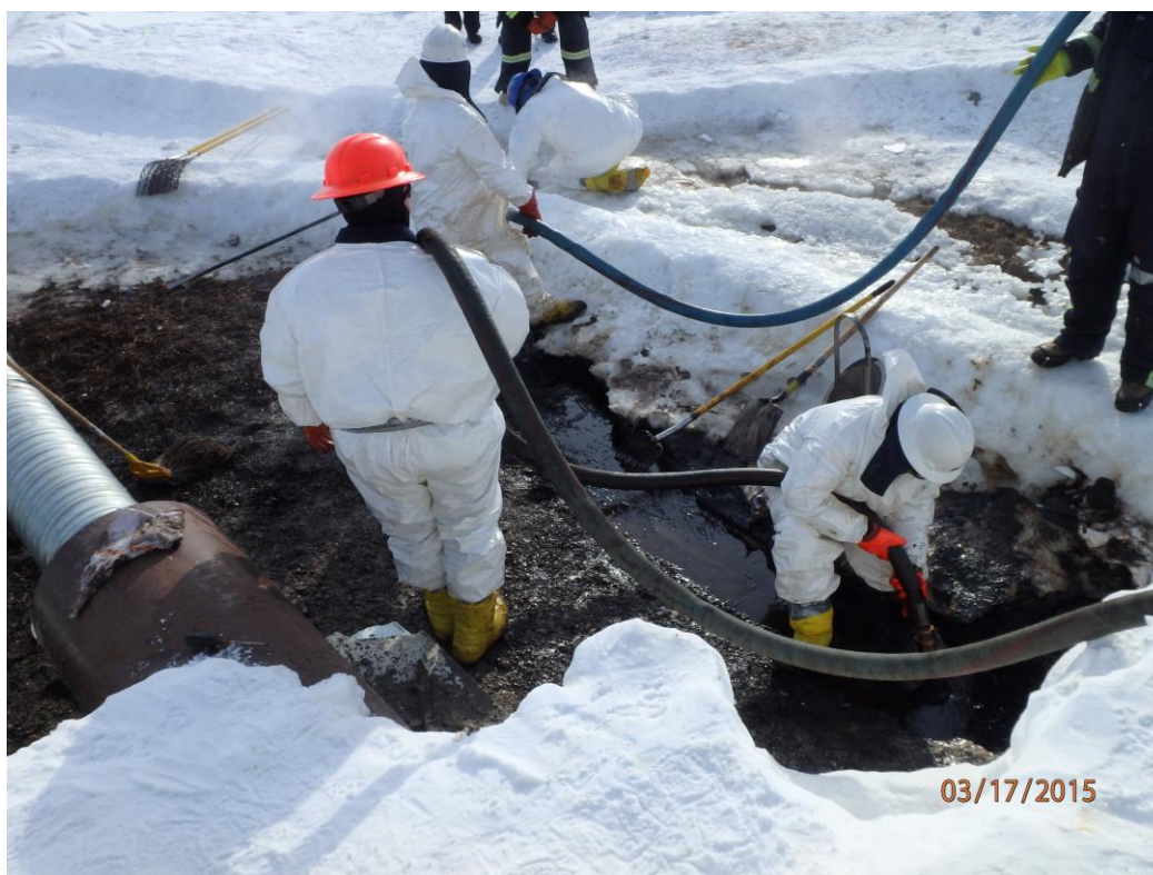
Figure 1. Tundra flood/flush and recovery operations to recover released fluids.
