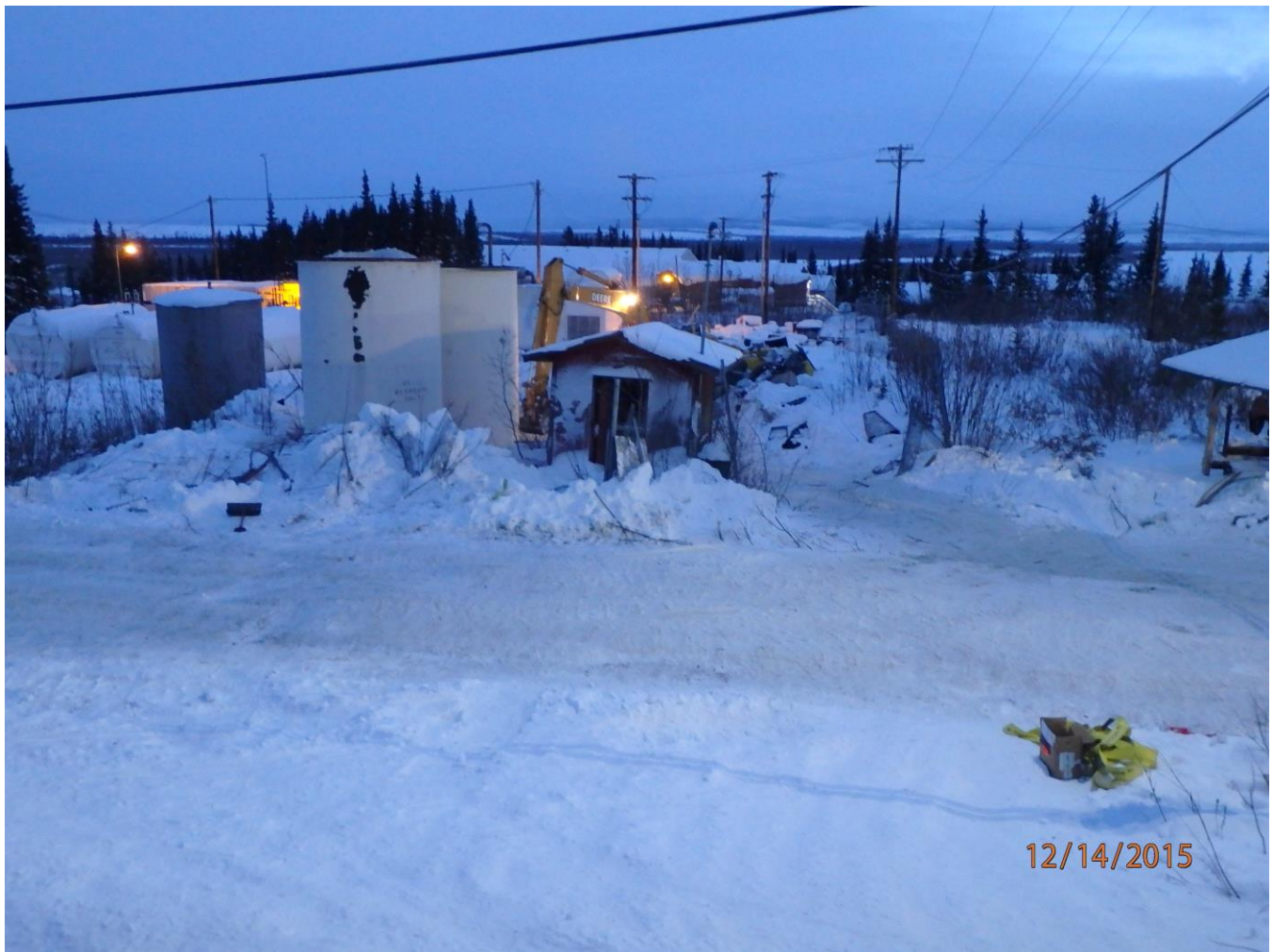
Figure 2. Backhoe moving contaminated snow into two vertical storage tanks for melting. [Photo: ADEC/John Ebel]
