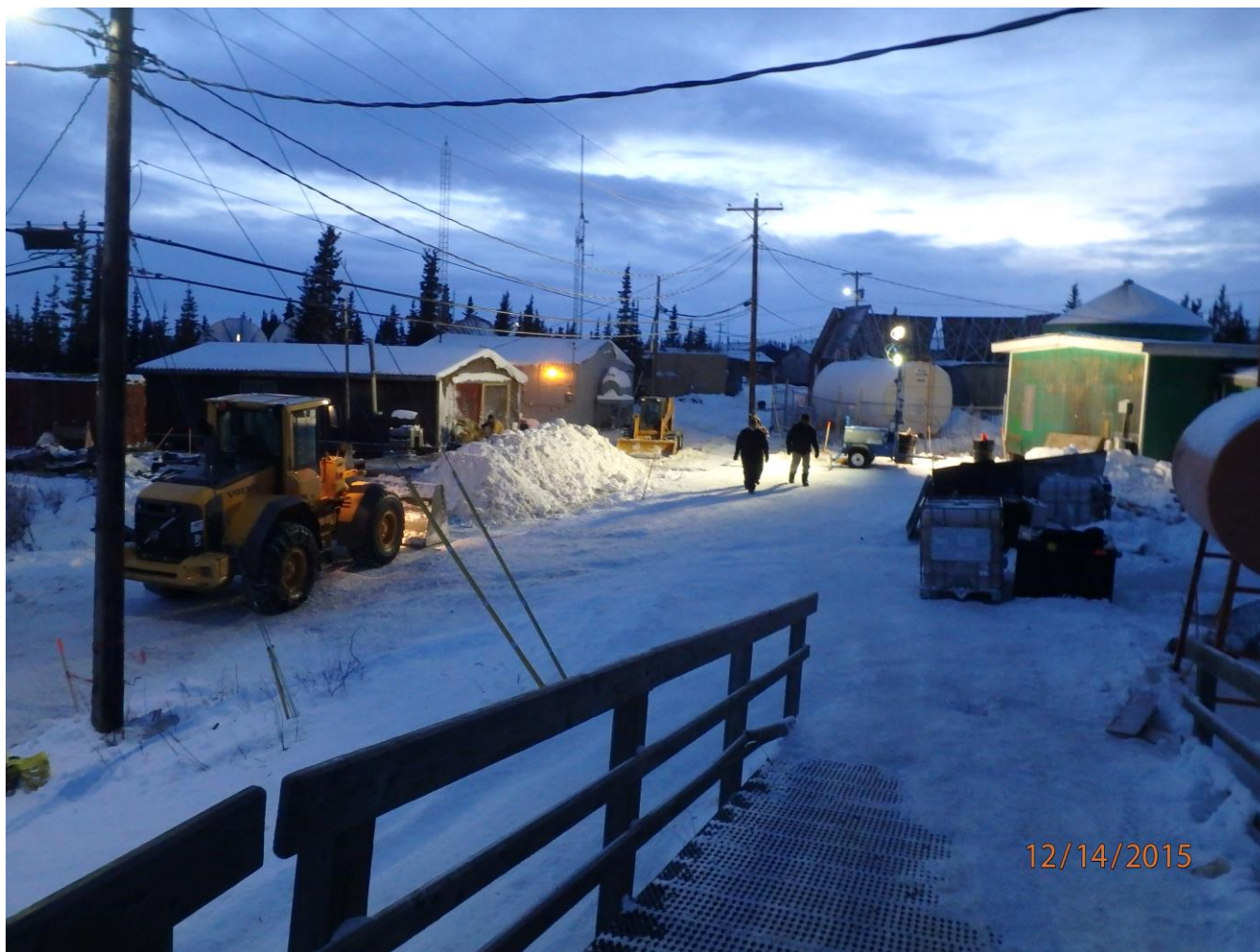
Figure 1. City tank is on right behind light plant; and the loader is moving contaminated snow from the “hot zone” to the vertical tank melting area. [Photo: ADEC/John Ebel]
