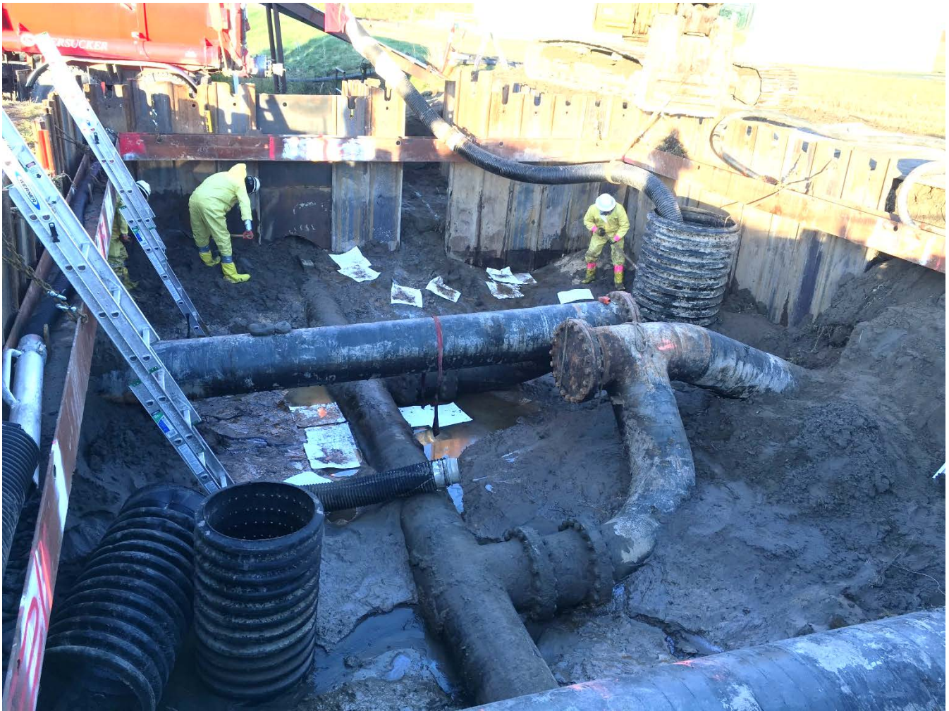
Excavation activity at dig site 1, September 23, 2016. (Photo/ADEC)
