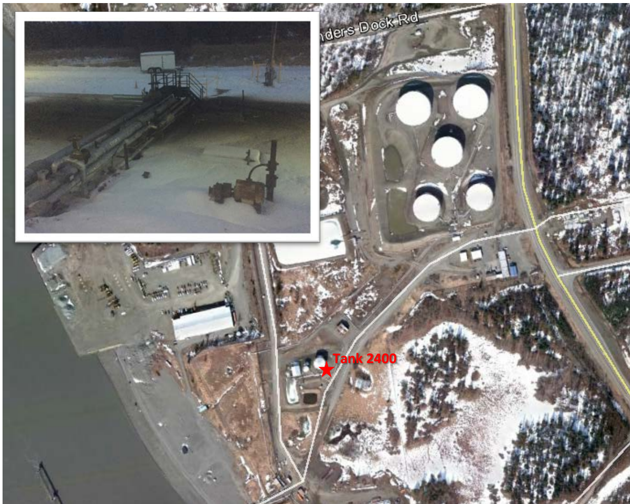
Spill location and photo of discharge, December 18, 2016. (Photo/Tesoro)
