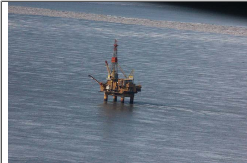
Platform A and mid-channel ice belt, facing west.
