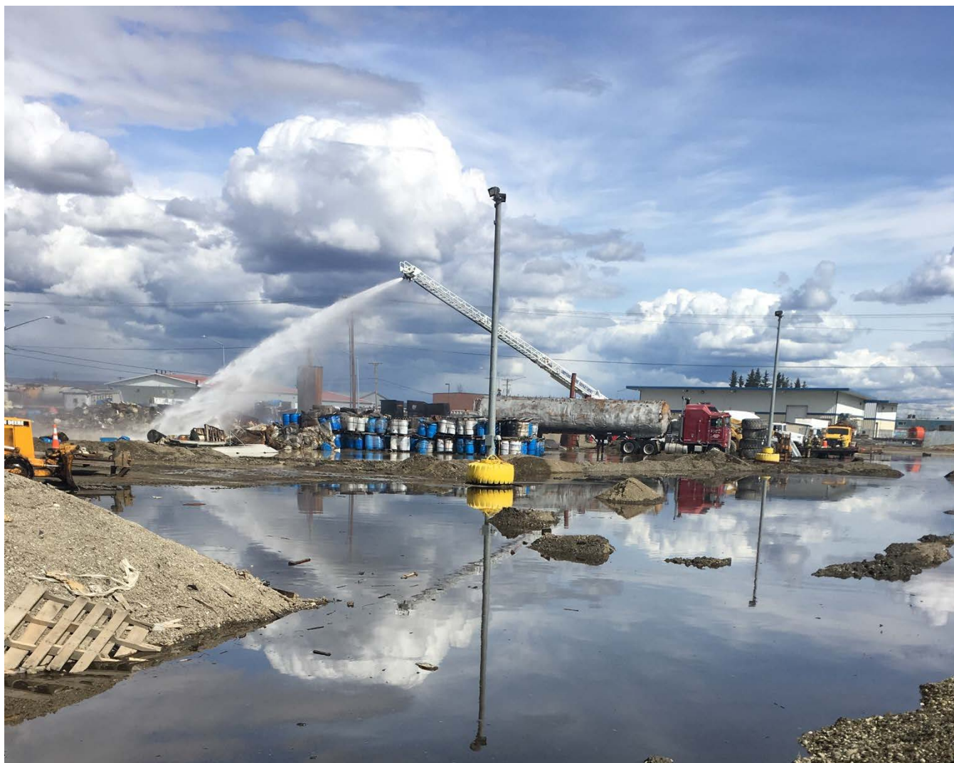
Figure 1. Fire crews work to put out the fire at the Bloom Enterprises, Inc. property on May 9, 2017. [Photo: ADEC]
