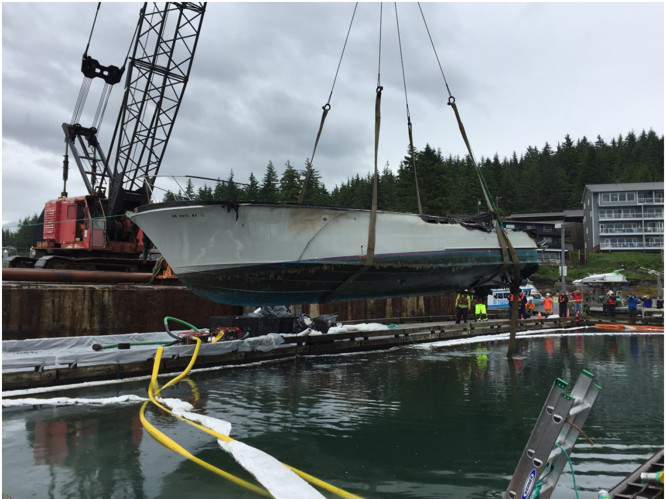
Raising of the M/V Whimsea onto Trucano's crane barge, pictured in the background. (Photo credit: ADEC; June 30, 2017).
